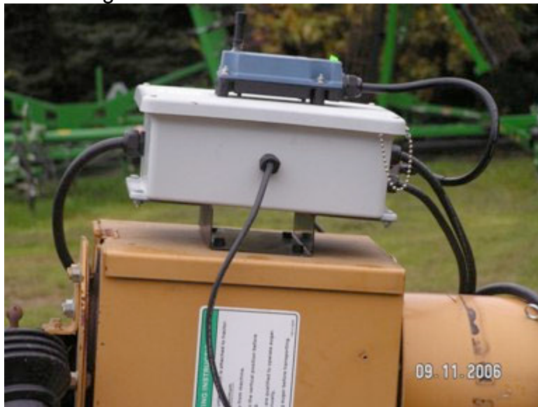
Receiver is now mounted inside the control box.
